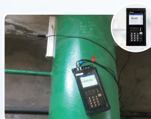
Measurement on a 0.4m Pipeline
